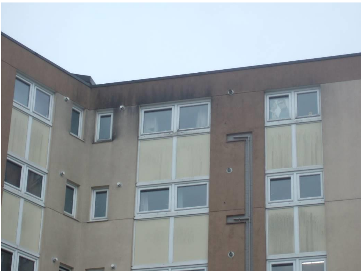
South elevation showing gas riser
