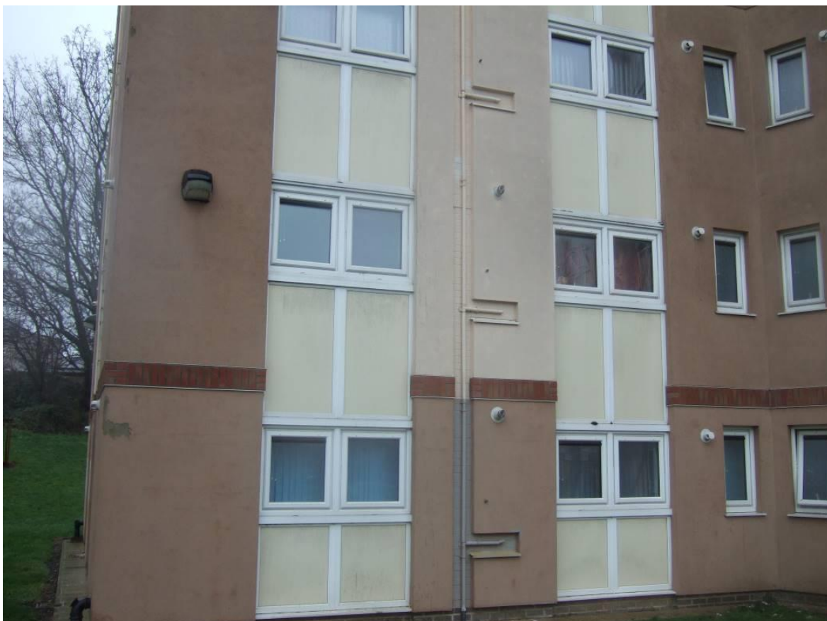
East elevation – showing gas riser
